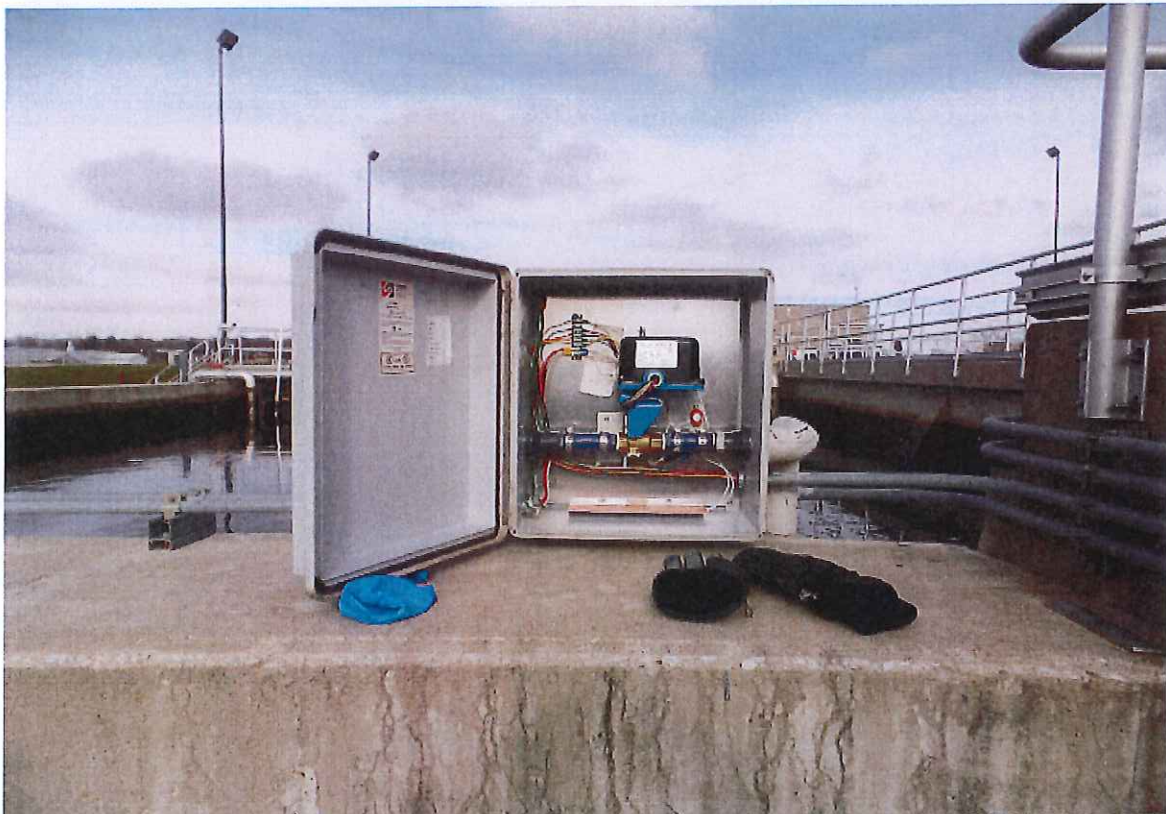
SBR 1 Decant Vent Valve East Side; Exhaust Side of Vent Plugged with Ice
