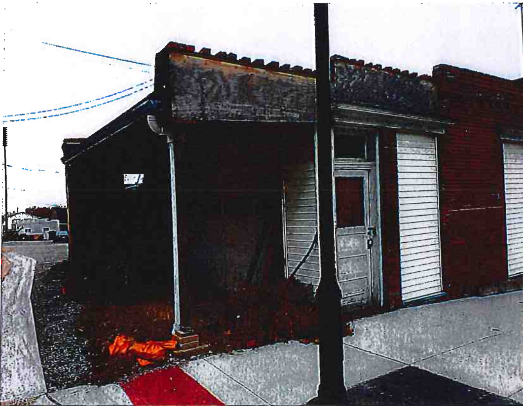
1st Street Garage
