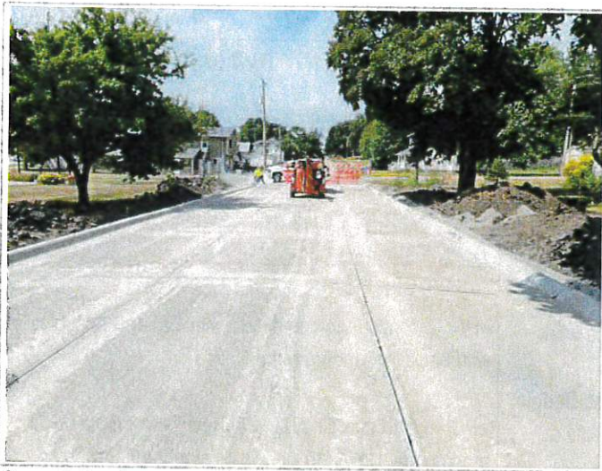
Concrete has been poured, cut and sealed from 2nd & Ella around to 2nd & Rose Streets
