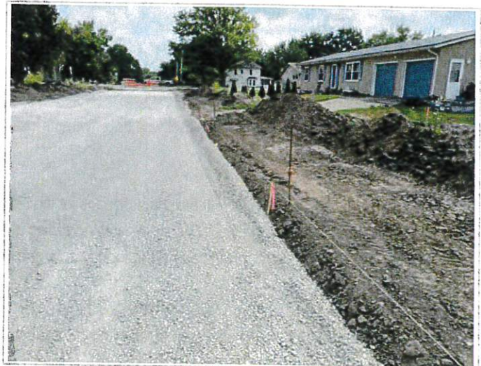
Streb has string-lines set throughout the rest of Phase 1 as they prep for upcoming paving
