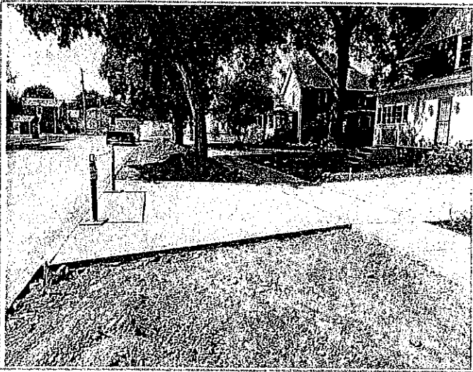
Sidewalks and driveways have been poured along both the north and south sides of 2nd Street
