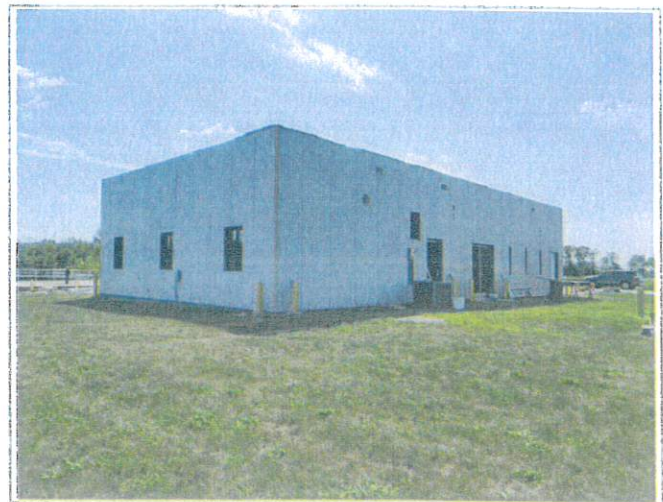
Overview from the NE corner shows progress of panel installation.
