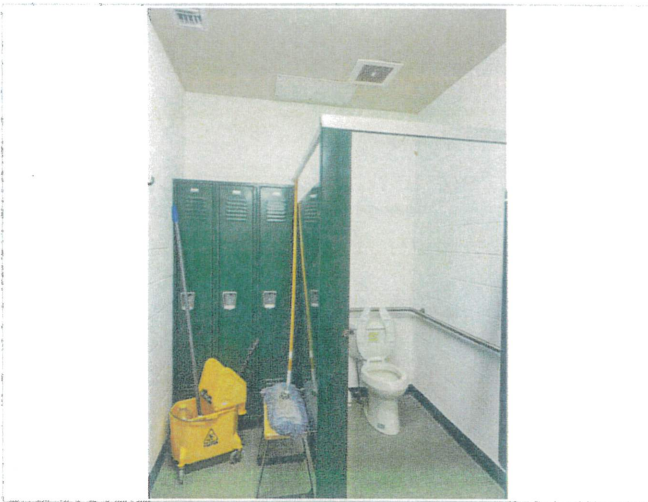
Restroom paint application is complete
