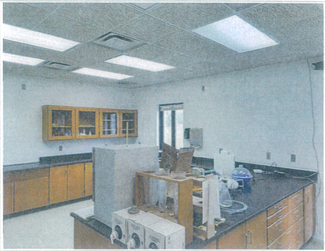
Overview of the Laboratory shows all the walls have been painted
