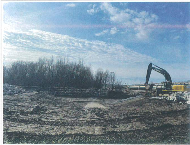
Looking South down boat ramp.
