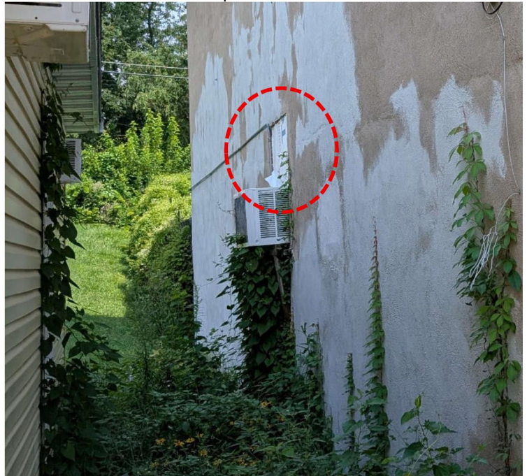
Photo 2: 41W, area to be patched with stucco
